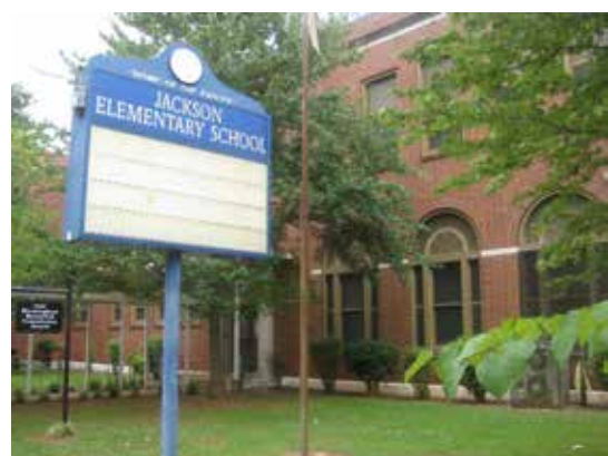
STONEWALL JACKSON ELEMENTARY SCHOOL IN THE WEST END COMMUNITY IS CURRENTLY CLOSED, BUT IS IN A PRIME LOCATION TO SERVE AS A COMMUNITY RESOURCE. SOURCE: RPCGB
