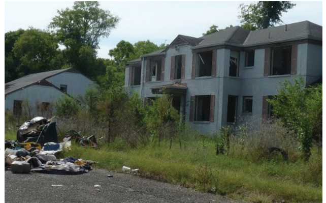
Larkway Gardens (Source: City of Birmingham)
