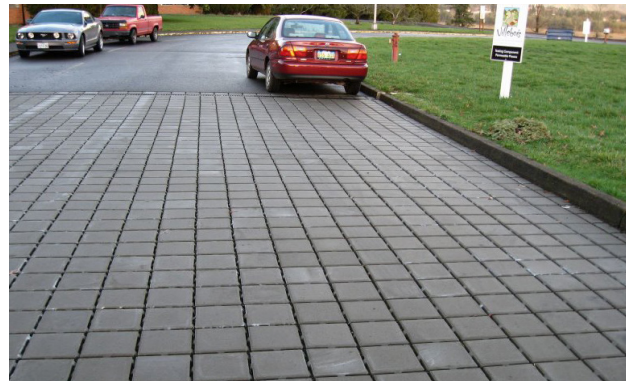
Permeable Pavement (Source: Environmental Protection Agency )
