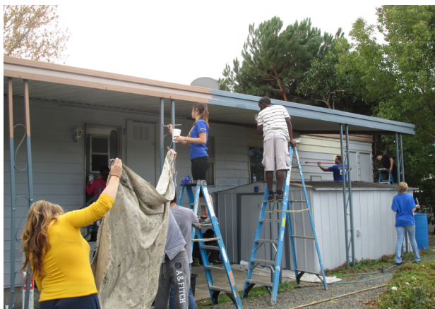
Volunteers rehabbing a house (Source: Habitat for Humanity Riverside)
