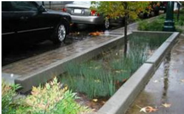
Planter Box (Source: Environmental Protection Agency )
