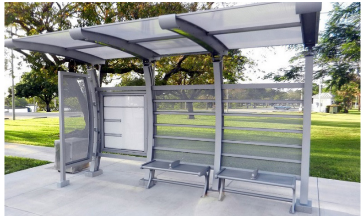
Bus Shelter (Source: Brasco )
