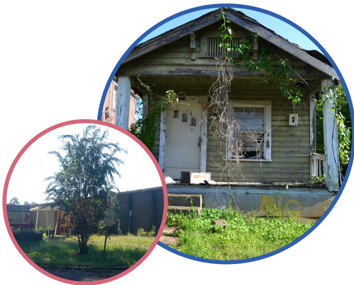
Above: Dilapidated house Left: A.G. Gaston School
