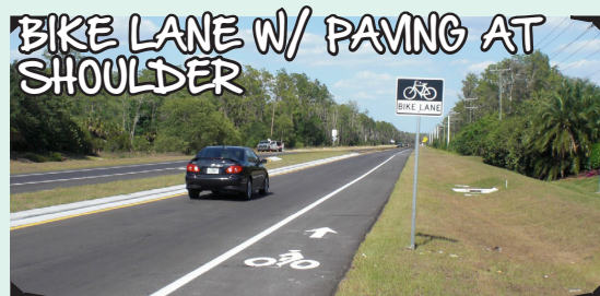
Image: Existing paved shoulder converted into a bikelane with signage and pavement (Source: bikewalklee.blogspot.com/ )
