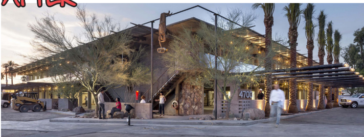
The Strip, an adaptive reuse development in Phoenix, Arizona was transformed from a tired building into a vibrant mixed use development complete with live work units, artists space, restaurants, and retail (Source: www.phoenixnewtimes.com/ )
