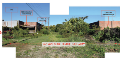
BEFORE / FACING EAST TOWARDS AVONDALE
