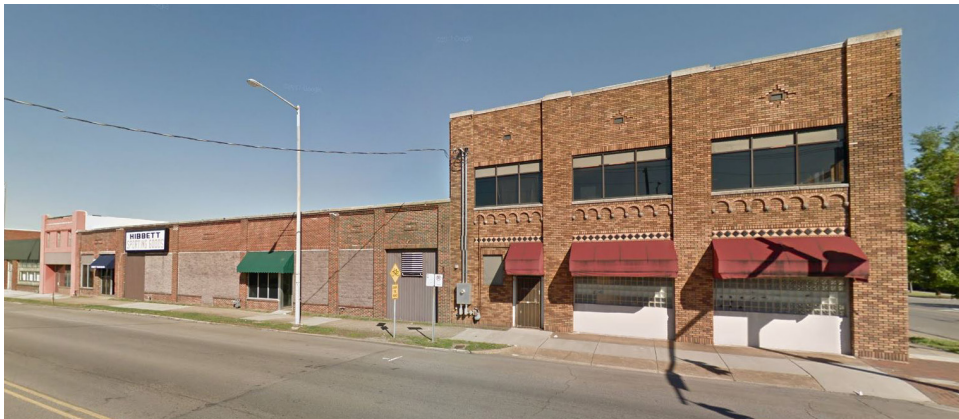
Left: Existing conditions at the northwest corner of 14th Street North and 1st Avenue North
