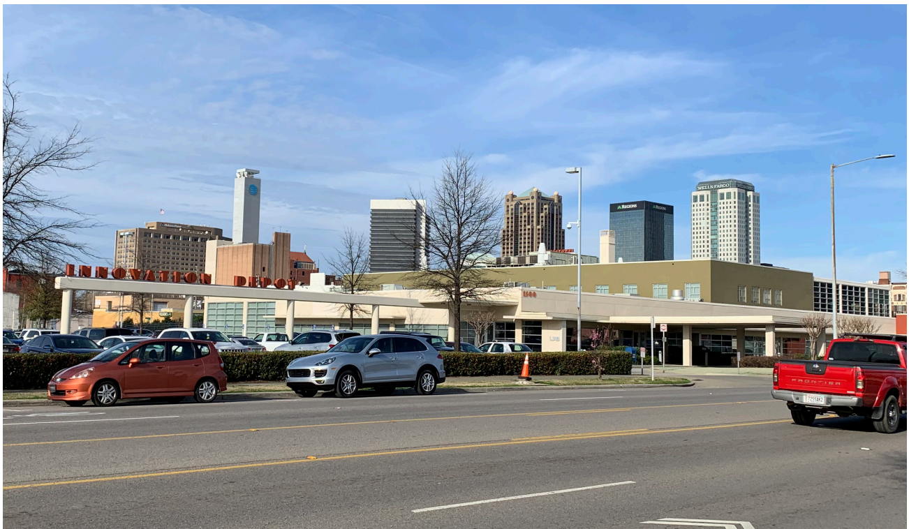
The main entrance of Innovation Depot as seen from across 1st Avenue North
