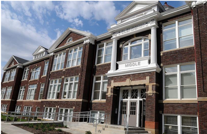
Left: Riverview at Clendenin School (Source: AU Associates)
