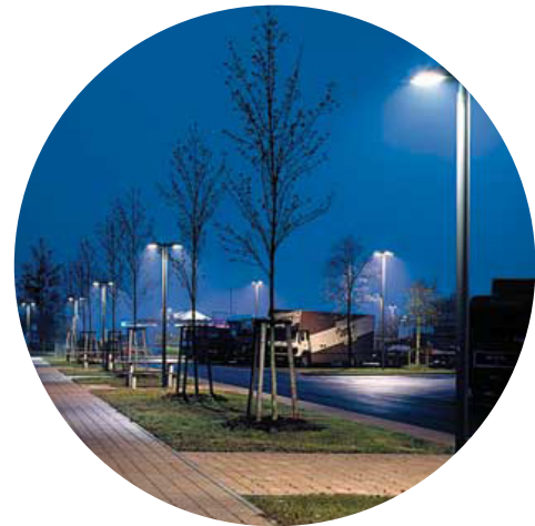
Adequate lighting, clear site lines, multiple viewpoints, programming, and creating pedestrian oriented landscapes + public spaces are all key elements of CPTED.
