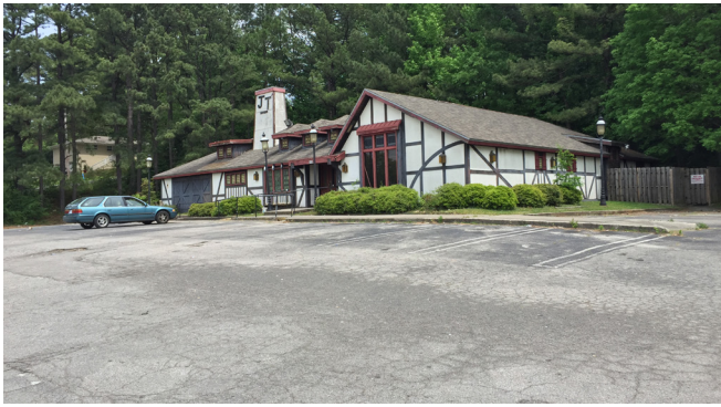
A vacant restaurant along Parkway East.
