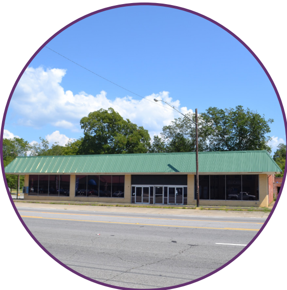
8515 1st Avenue North
