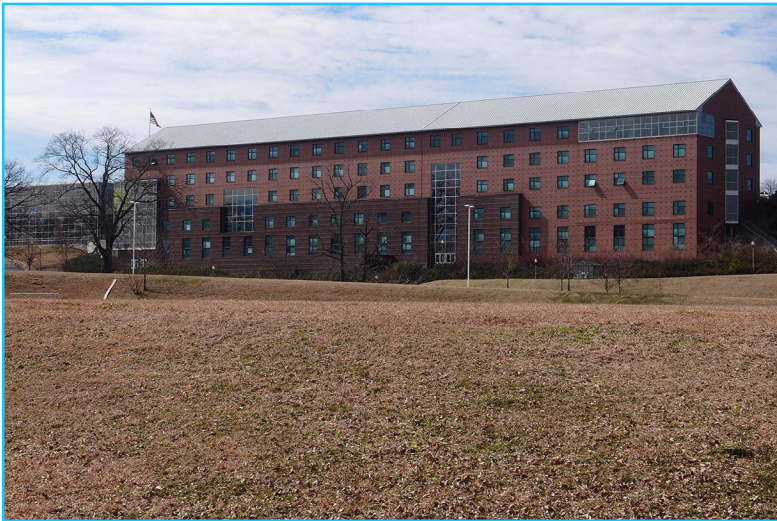
George Washington Carver High School, located in the North Birmingham Neighborhood (above)
