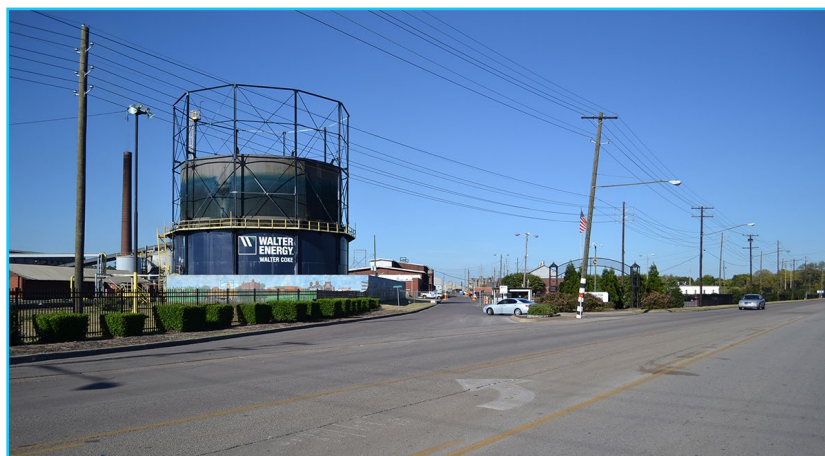
Walter Coke plant, opened in 1920 (above)
