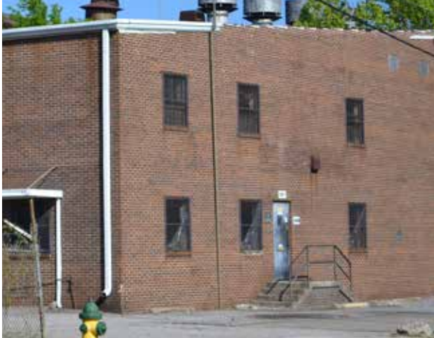
Trinity Steel Plant
