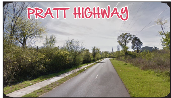
Construct sidewalk on right side of street.
