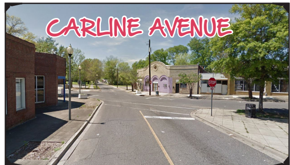
Repair cracks and holes in sidewalk.
